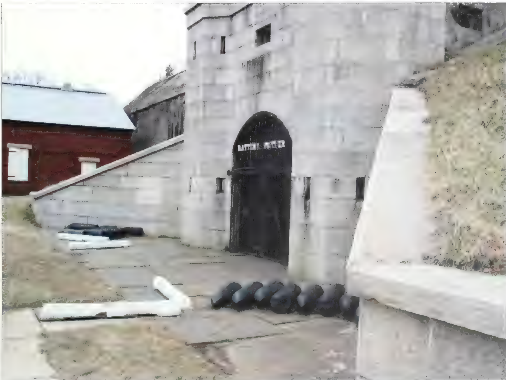
Figure 5.58. View looking north at defensible main entry, Battery Potter. The main entry is through an arched opening flanked by defensive stone towers. Each tower had gun loop slots so machine guns could fire on potential attackers. The entry facade resembles a castle and was constructed from granite blocks salvaged from Sandy Hook's Civil War-era fort (Olmsted Center, January 2009).
